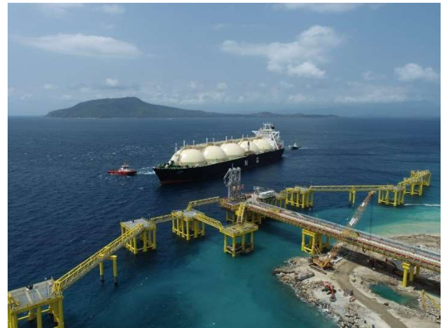
LNG terminal at Ilijan Power Plant in Batangas.
